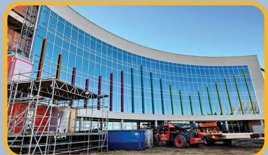
Bethany Children's Health Center Expansion, Oklahoma City, OK
